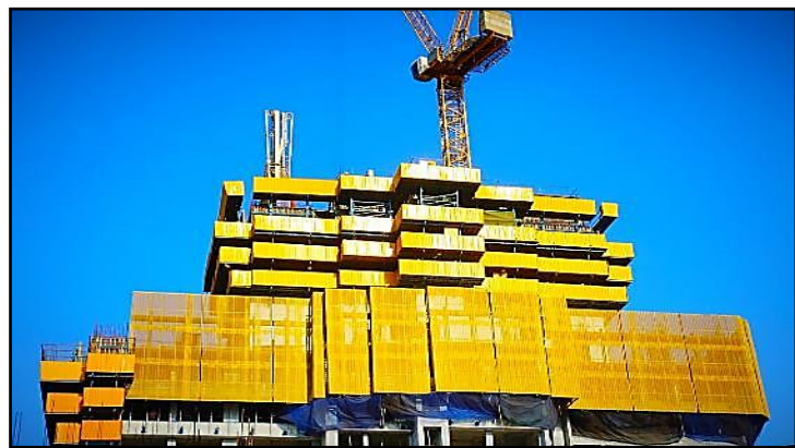
Safety Screens around the floor on which work is in progress
